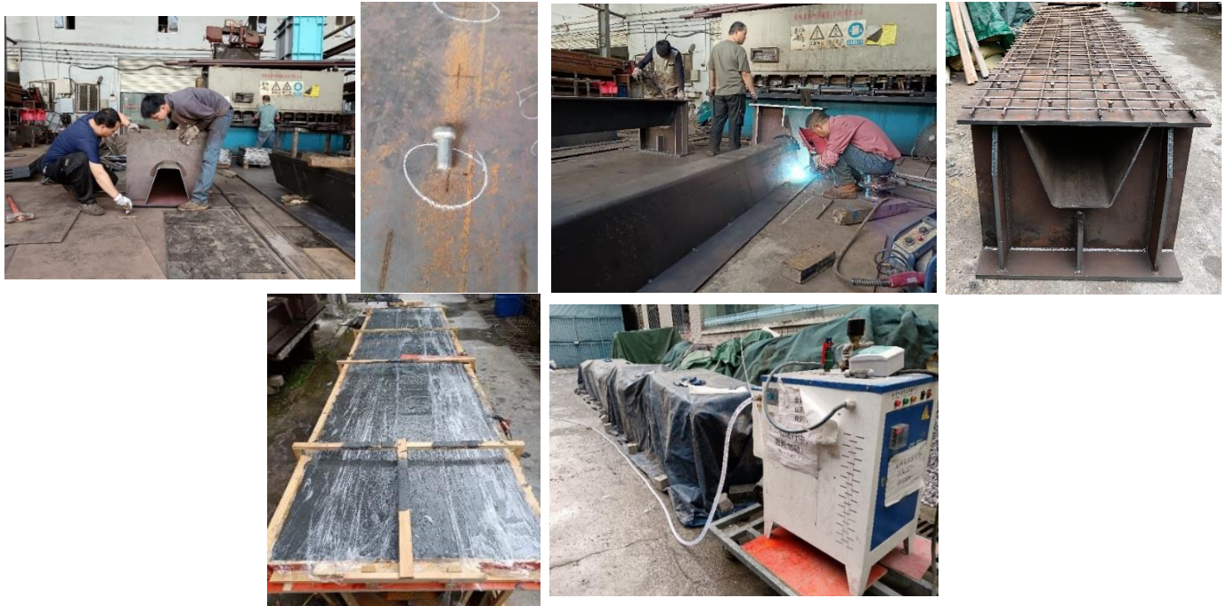
Figure 5. Fabrication processes of the specimens and steam curing of the slabs.
